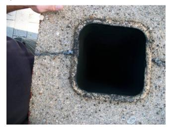
10. Fireplace chimney flue is filled with creosote/debris – recommend having chimney sweep clean and inspect flue liner
